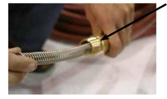
Once you have established which end has a slightly larger circumference, feed the other end, the narrow side inside your hose before installing the hose onto the reel.
